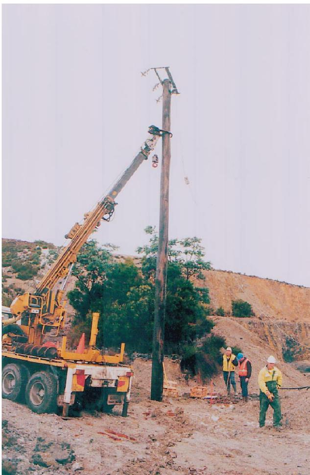
**Figure 2.** Assembly of one of the power poles near the gravity plant, Comstock Mine, Zeehan
