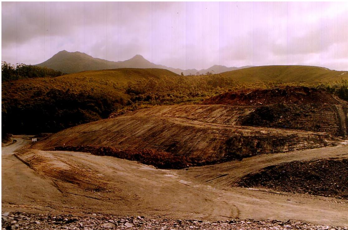
**Figure 3.** Rehabilitation of the Central Waste Dump (CWD). Clay is covered and compacted over acid producing material. Photograph taken looking to the NW.
