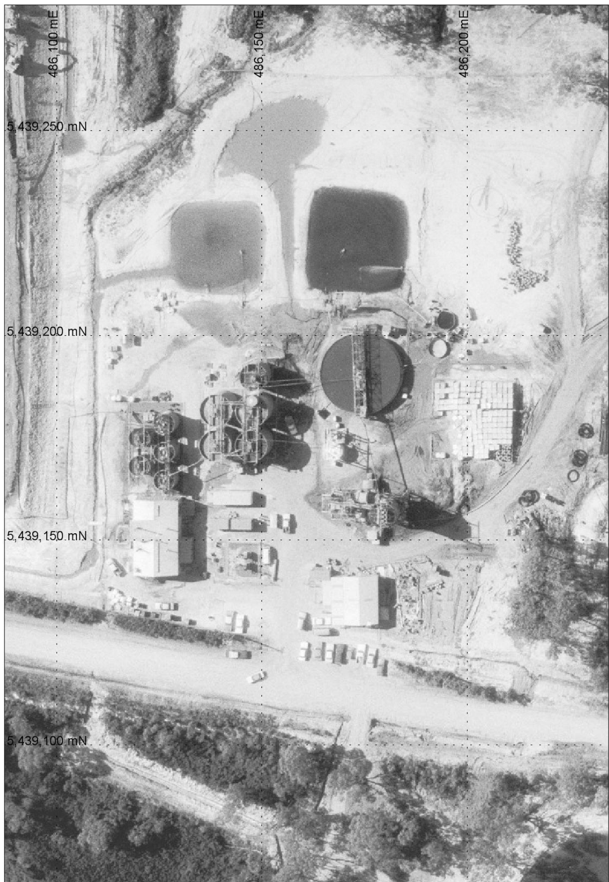
Figure 2 Golconda plant site October 1986.
