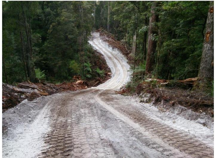
Topsoil removal: strippings downslope for silt control
