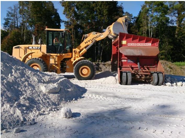
**Oversize will be broken down and re-screened**
