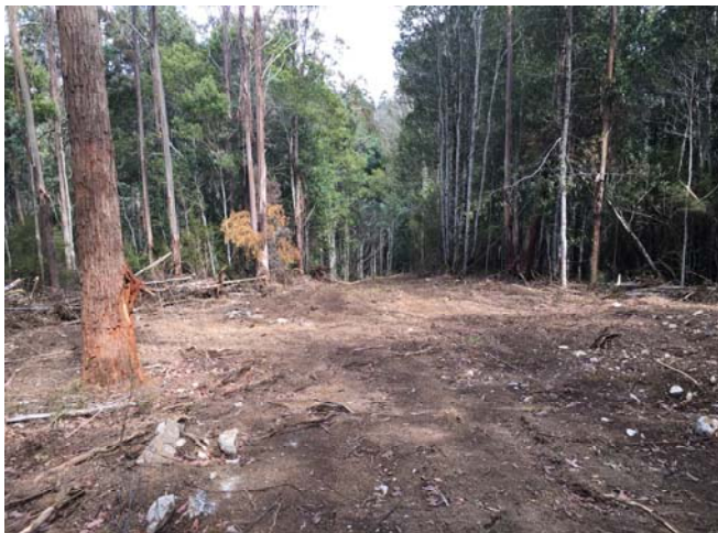
Grass verge of Roberts Road leading into the existing track which was refurbished for site access to conduct drilling
