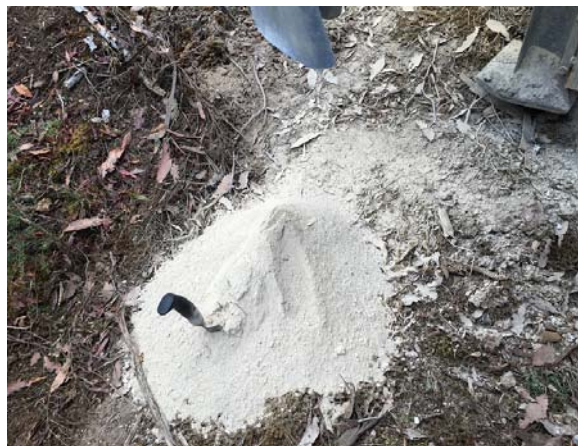
Limestone powder adjacent to the percussion drill rig
