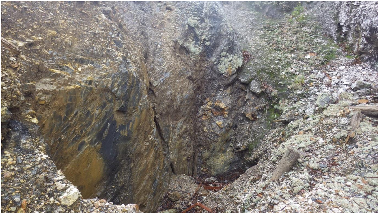
figure 3.5: Murrays Reward shaft now collapsed.
