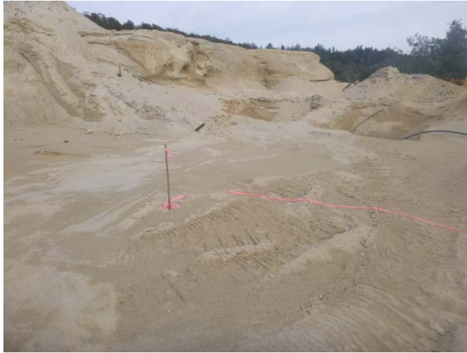
Photo 3. Drill Site for MDD003
