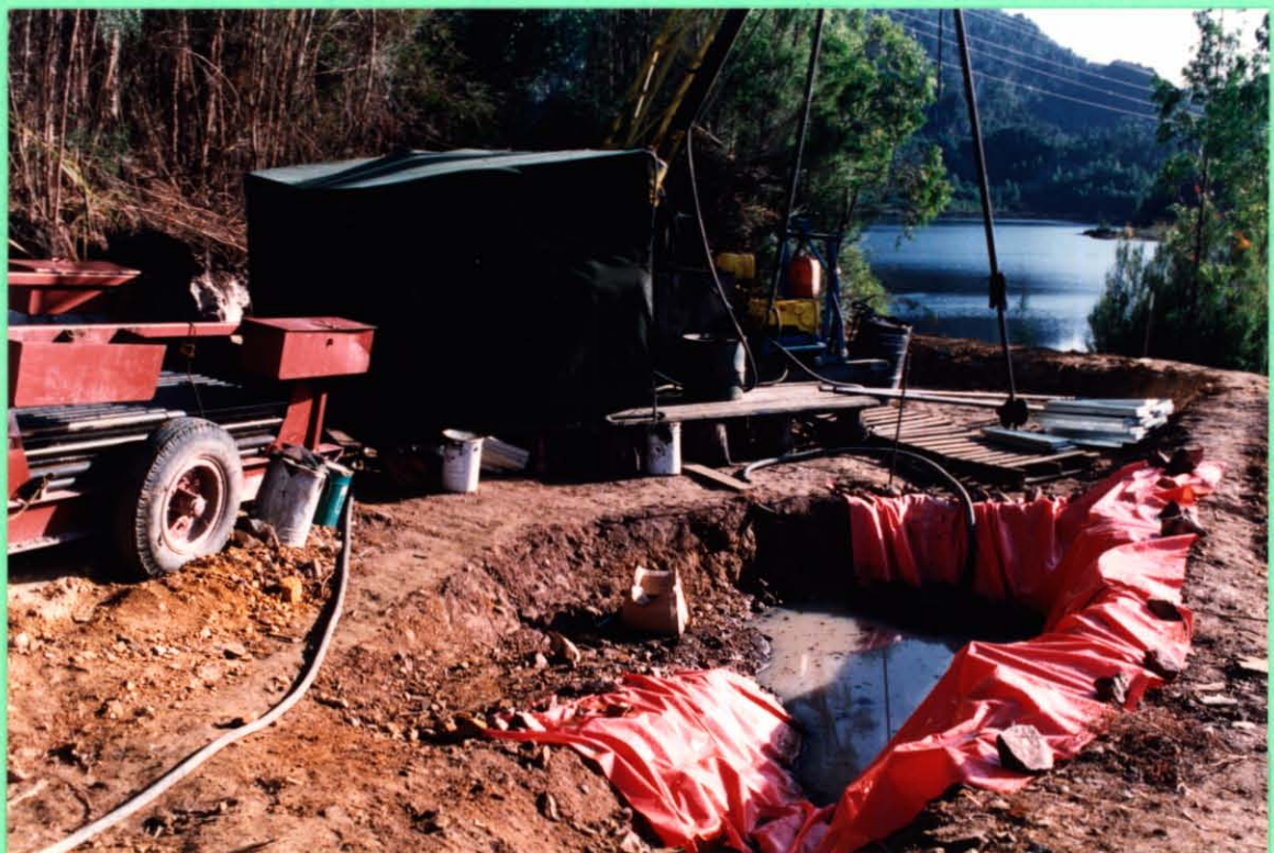
Plate 2 BY2 drillsite, Showing perimeter bund and sump for temporary effluent storage
