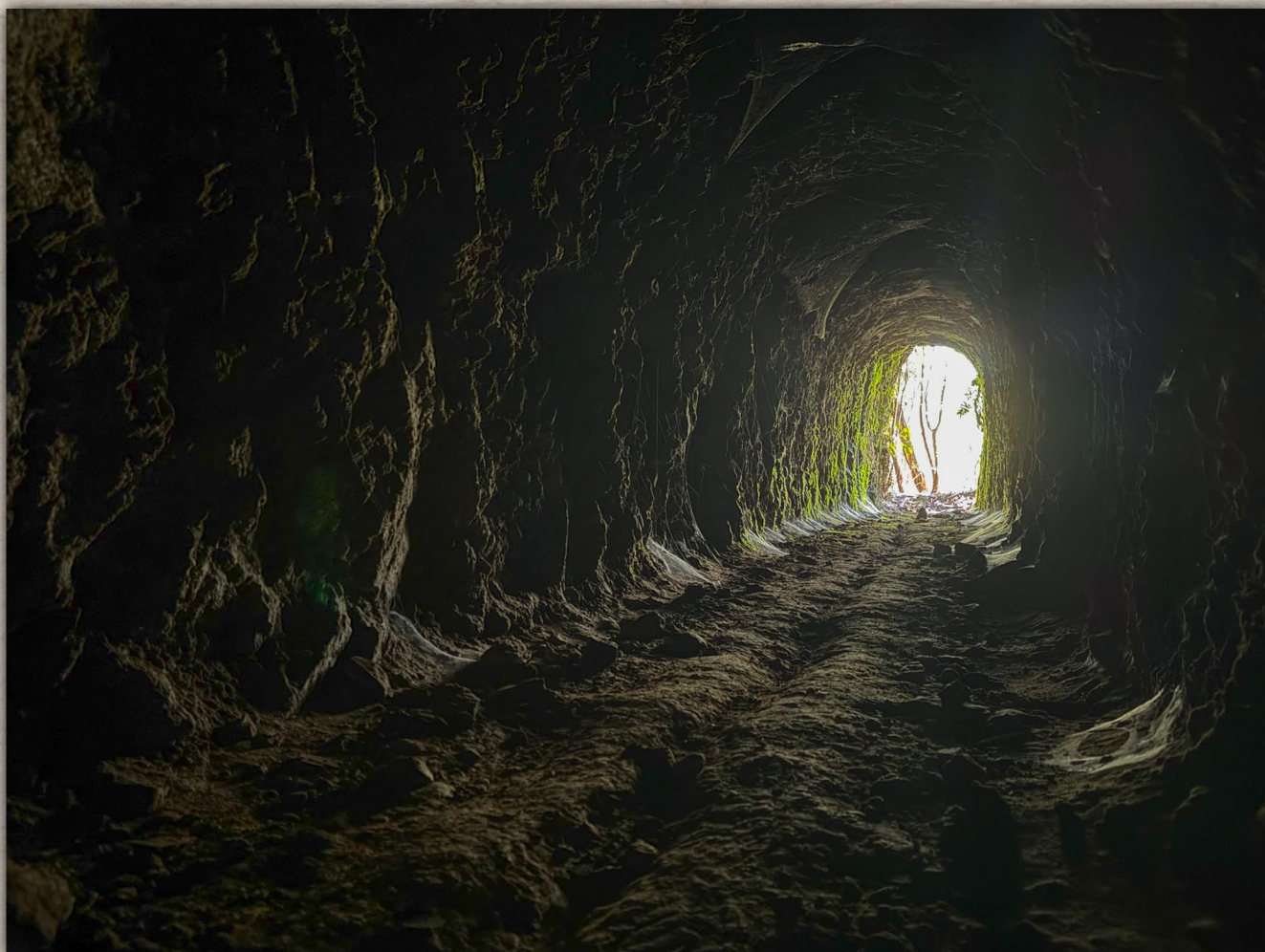
Slaters Tunnel (120ft) midway, looking outside
