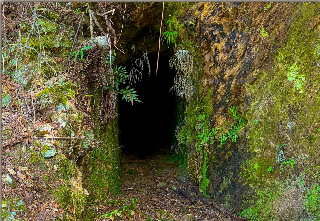
Portal to Slaters Tunnel (120ft)
